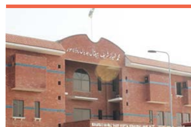
61 Muhammad Shahbaz Sharif Hospital, Bedian Road, Lahore BED General Hospital
